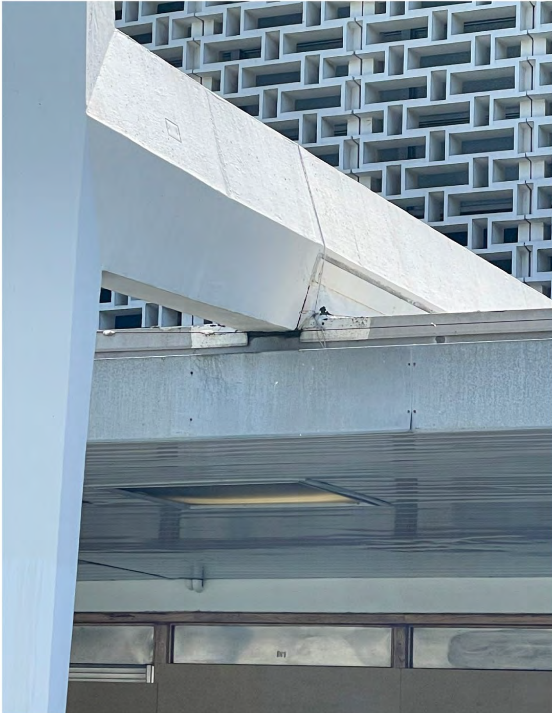
Figure 11. Geometric pylon, floating canopy, brise-soleil (view east). Image: Nina Fresco, 2023
