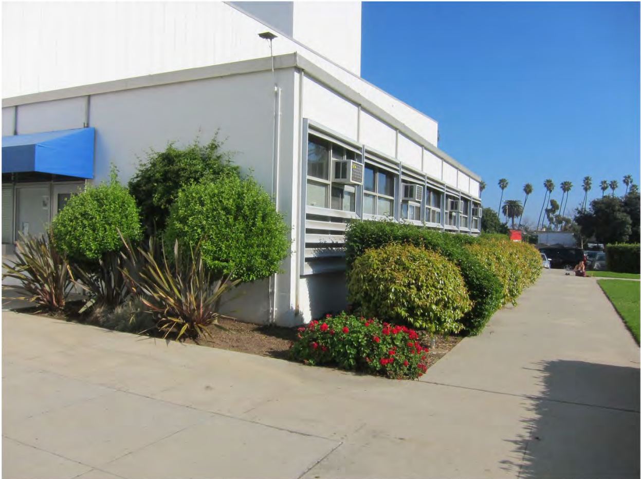
Figure 19. West Wing louvered windows (view east). Image: Nina Fresco, 2014
