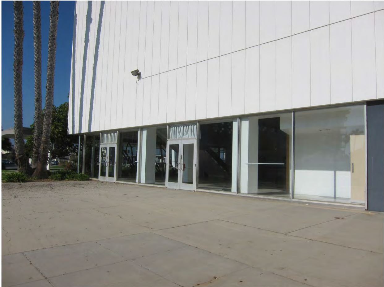
Figure 12. West Patio, scored concrete volume over glass-enclosed lobby (view north). Image: Nina Fresco, 2014
